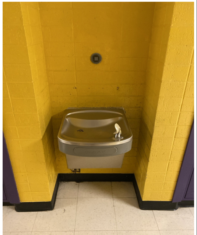
2/6/2024 - 1301-19 - Middle School - Outside Room 119
