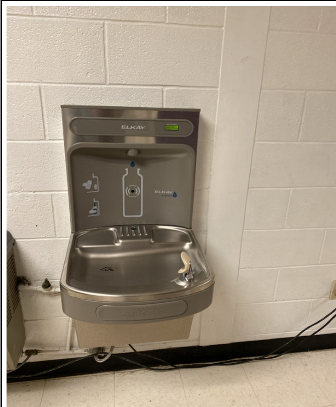
2/6/2024 - 1301-24 - Middle School - Outside Girls Restroom-Right
