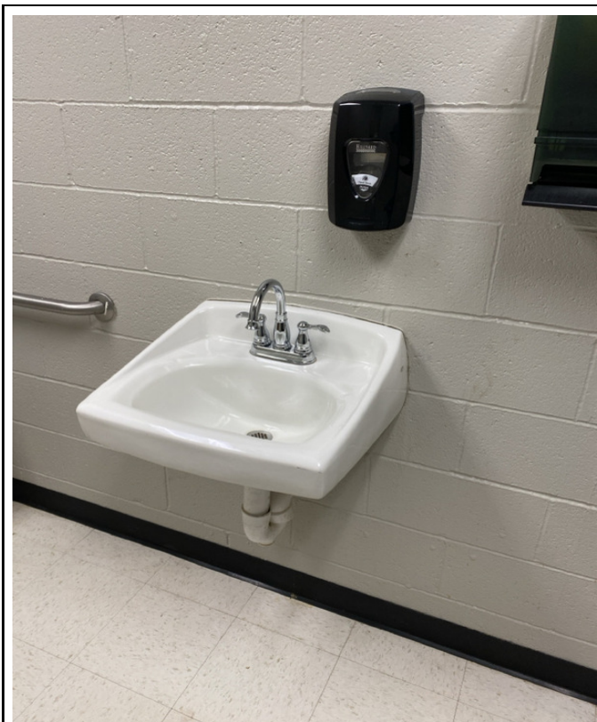
2/6/2024 - 1301-32 - Middle School - Art Room- Restroom
