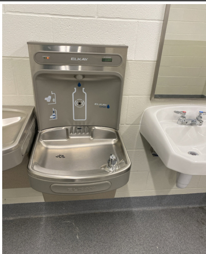
2/6/2024 - 1301-9 - Middle School - Boys Locker Room-Right
