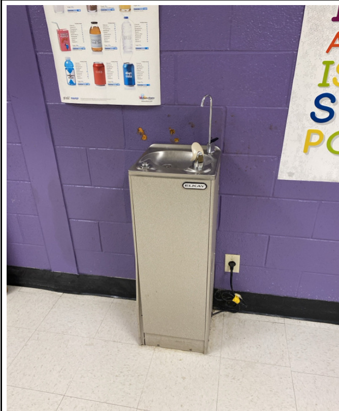
2/6/2024 - 1301-28 - Middle School - Cafeteria
