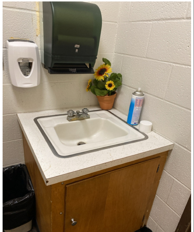
2/6/2024 - 1301-17 - Middle School - Nurse's Office-Hall Restroom
